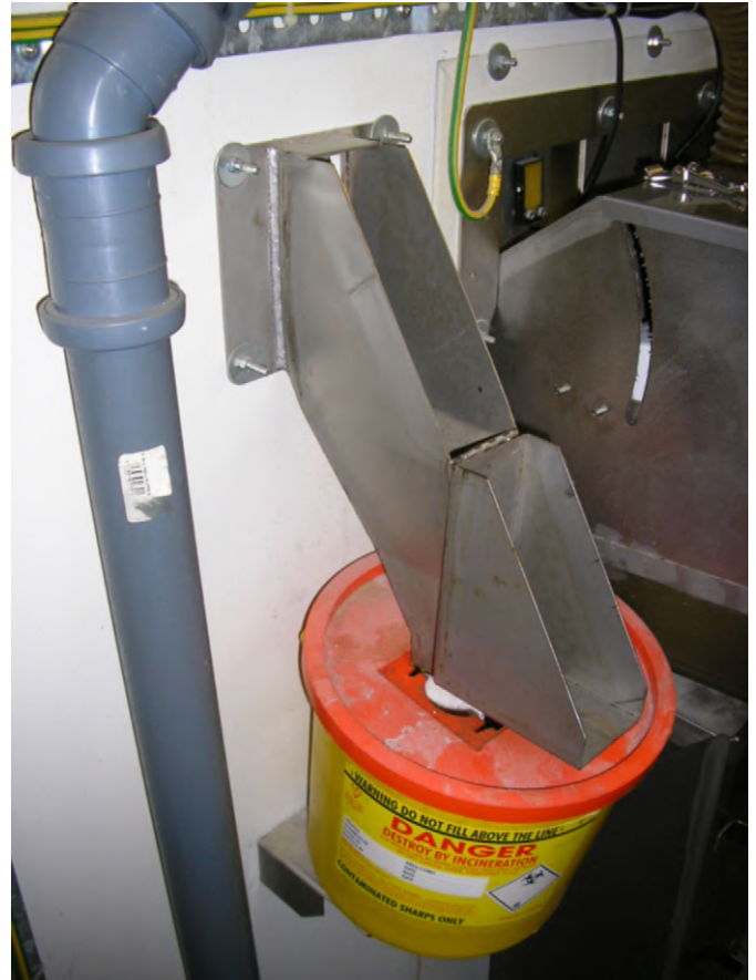
Fig. 3. Dedicated chute for sharps (rear of unit).
